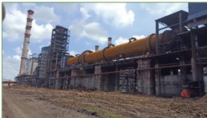
Figure 37: View of rotary kiln in DRI industry
